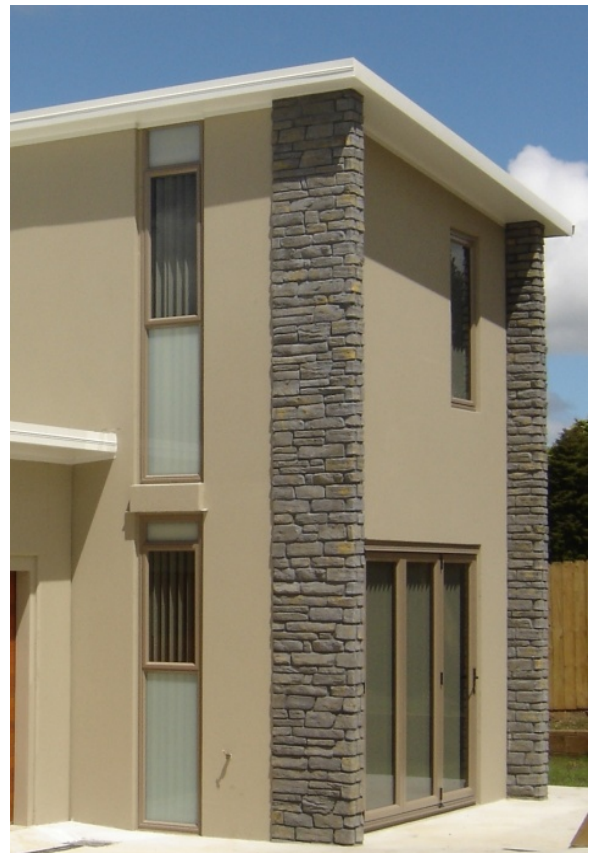
Thin stone veneers glued to Litecrete panel surface
