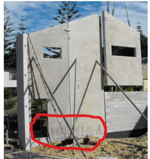
Option 1: bent starter bars
