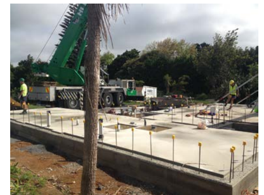
Option 2: Starters for Drossbach connection
