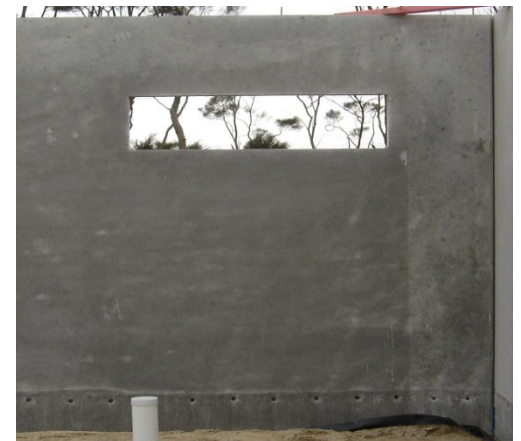
Option 3: Reid cast-in steel inserts
