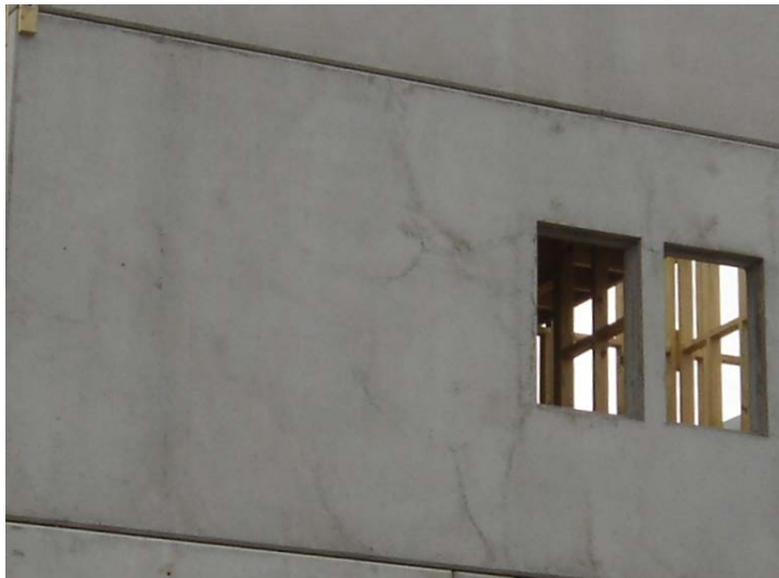
Photo shows typical surface figuring on a Litecrete panel.
