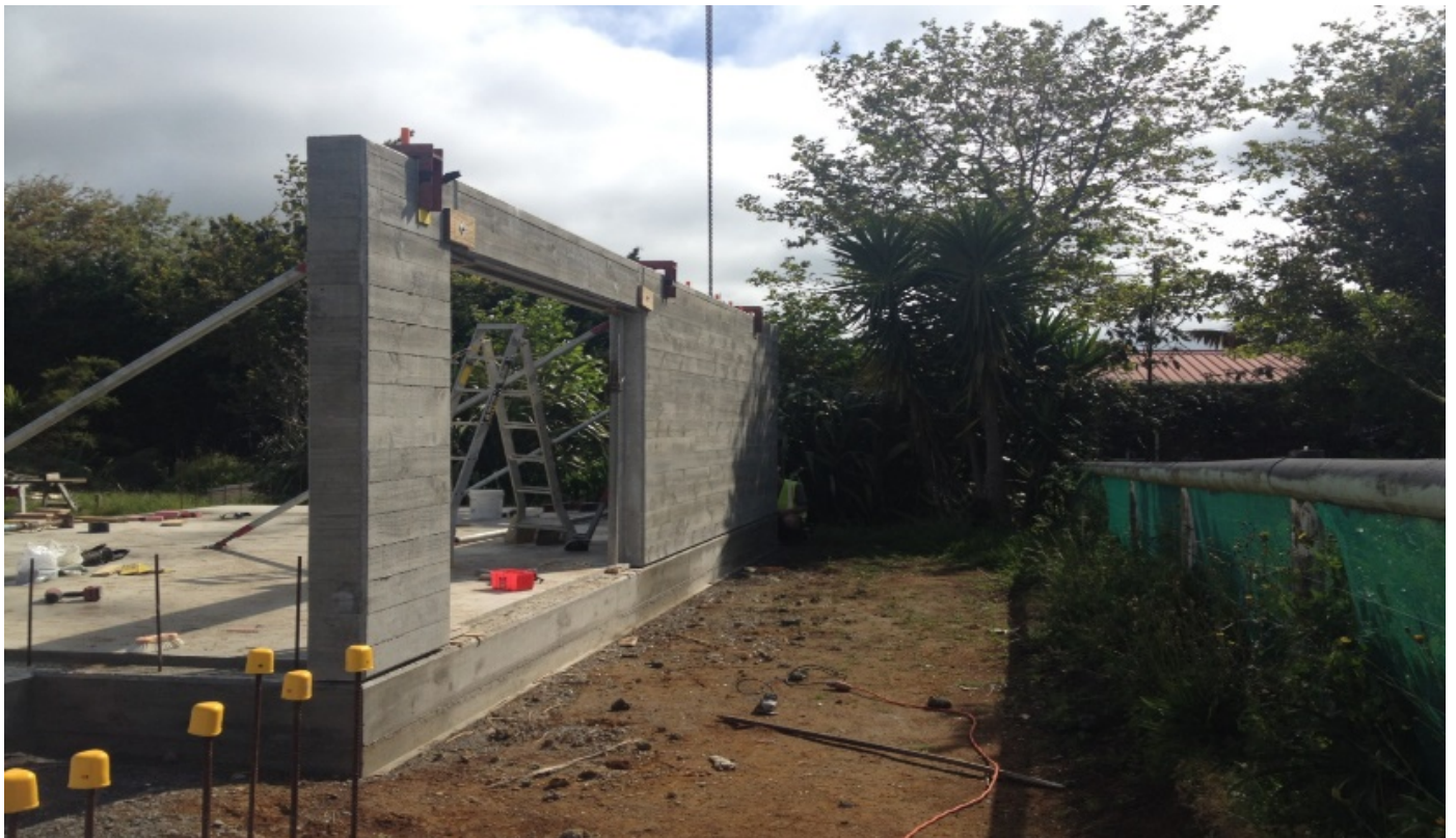
Rough-sawn timber finish on Awhitu beach house panels
