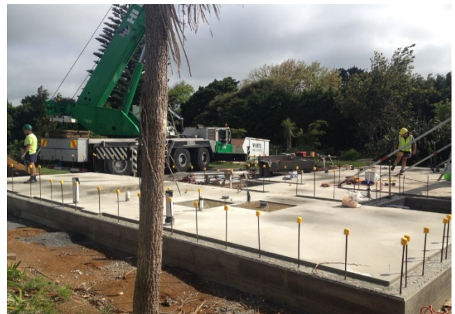
Photo shows the rebate and starter bars protruding from slab
